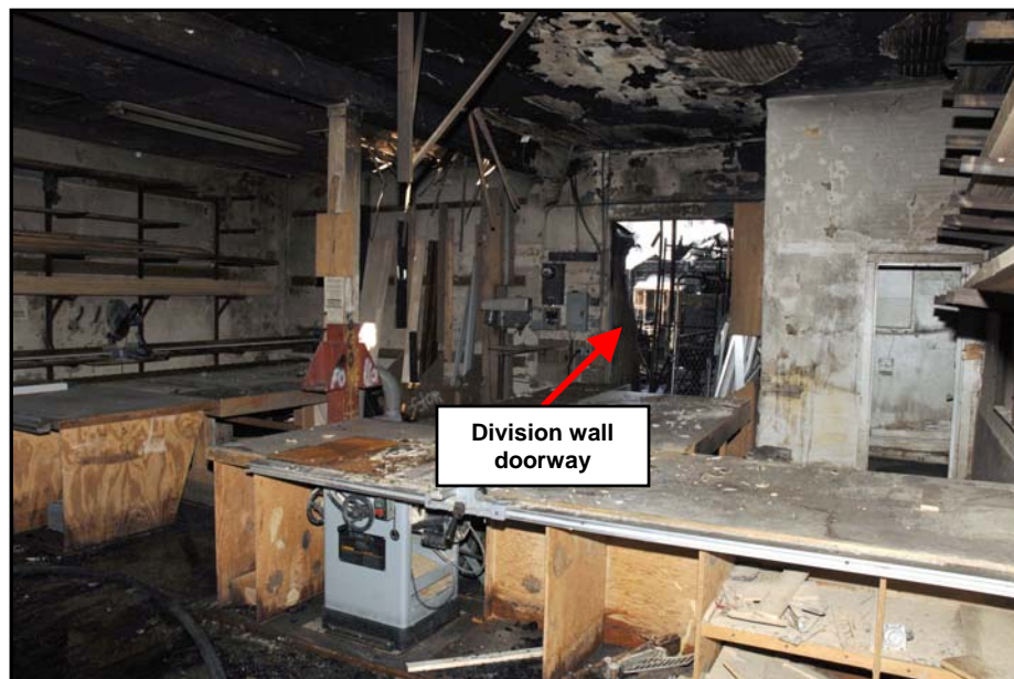
View of structure from "D" fire attack entry
