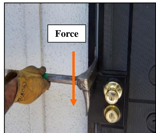
Photo 7: Leveraging down against the door frame will cause the door to flex enough to clear the deadbolt.
