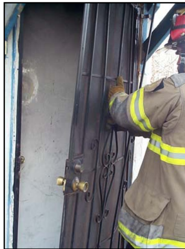
Photo 5: A quick jerk of the door will create enough flex to clear the deadbolt from the door frame.
