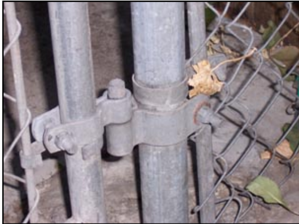
Photos 13 & 14: Attacking the hinge side of the gate is a quicker and easier method than trying to defeat a pad lock.
