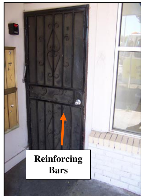
Photo 3: Reinforced security door.
