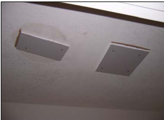
Photo 5- Cover all openings in the ceiling with sheetrock.
