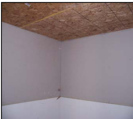
Photo 13- Reinforce burn corners with extra layers of sheetrock and OSB.
