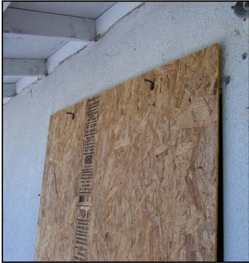
Photo 7- Using OSB and spikes for blow-out windows.
