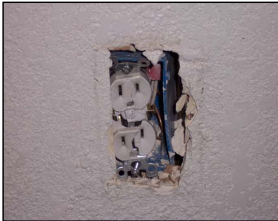
Photo 2- Remove all outlet covers.
