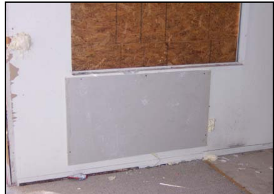
Photo 6- Cover all openings in the wall with sheetrock.
