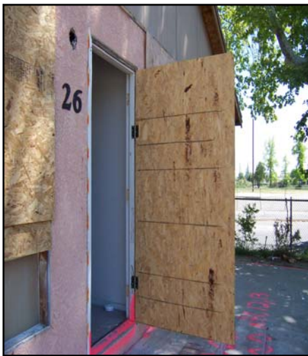
Photo 8- Using OSB and hinges to create a blow-out door.
