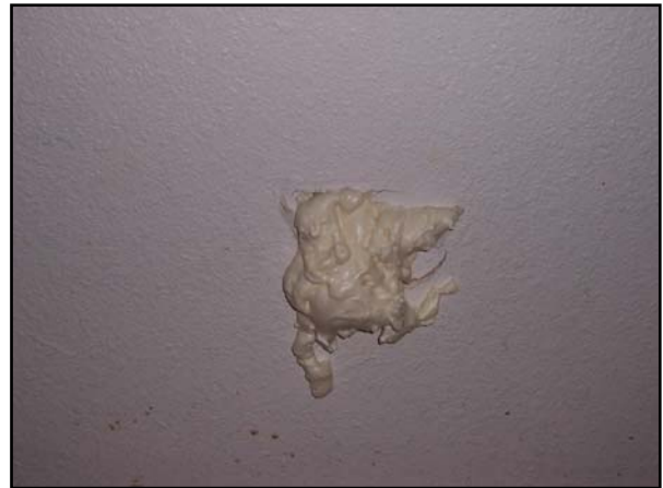
Photo 3- Allow foam to dry for 24 hrs.
