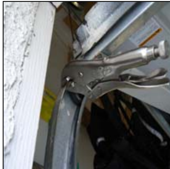
Photo-5: Using Vice-Grips to secure the door in place.
