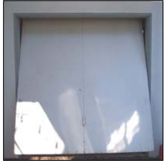
Photo-6: Typical Slab Door.
